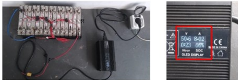
Fig. 9. Electric car battery charging trial in Polman
